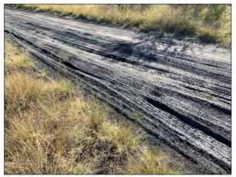
Figure 13: Unsealed track with coal reject / carbonaceous siltstone (2019)
