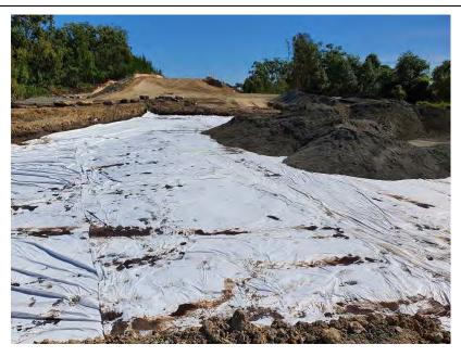
Photograph 26 – Showing placement of geo-fab, and stockpiled imported fill ready for placement, 20 Apr 2020.
