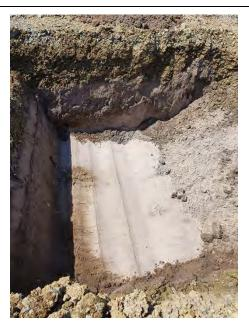
Photograph 23 – Test pit in Lot 108 showing profile of imported fill material overlying aeolian sands, 20 Feb 2020.
