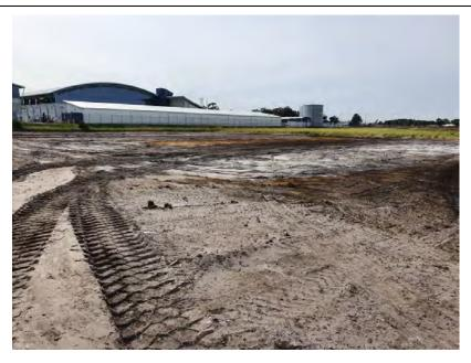
Photograph 27 – Showing Lot 101 and 102 after topsoil stripping and before placement of fill, 20 May 2020.
