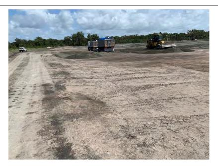
Photograph 21 – Placement of first layer of material on Lot 109, 17 Feb 2020.
